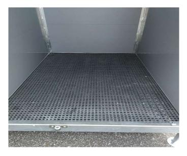
✓ FRP micro-mesh molded grating floor, which is additionally gritted to make it slip-resistant.
