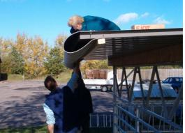
12. To make setting the screws easier, it is recommended to put another lath under the roof to support it.
